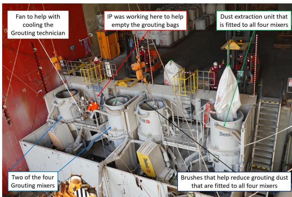
Grouting plant on vessel
